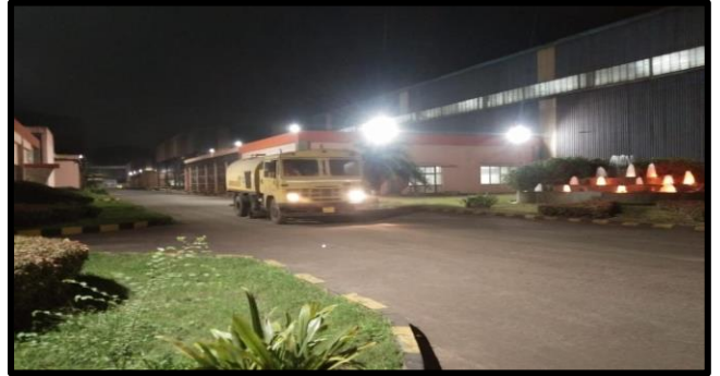
Regular Road repairing also being carried out.
